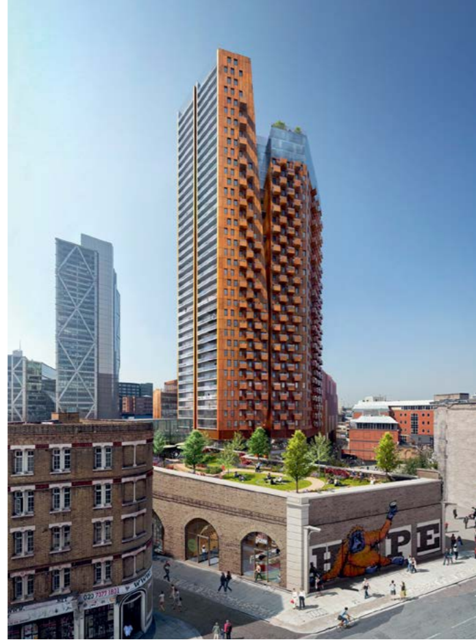
Project: The Stage Location: London, United Kingdom
