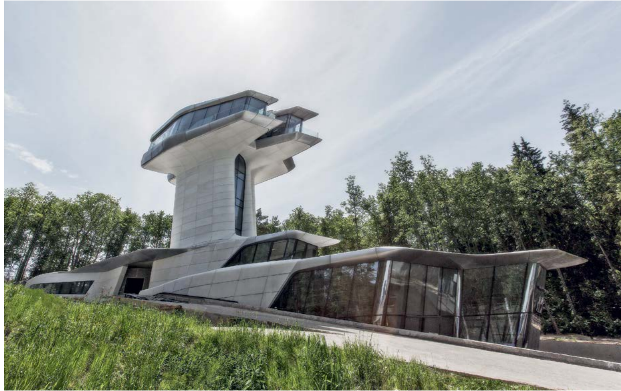
Project: Capital Hill Residence Location: Barvikha, Russia
