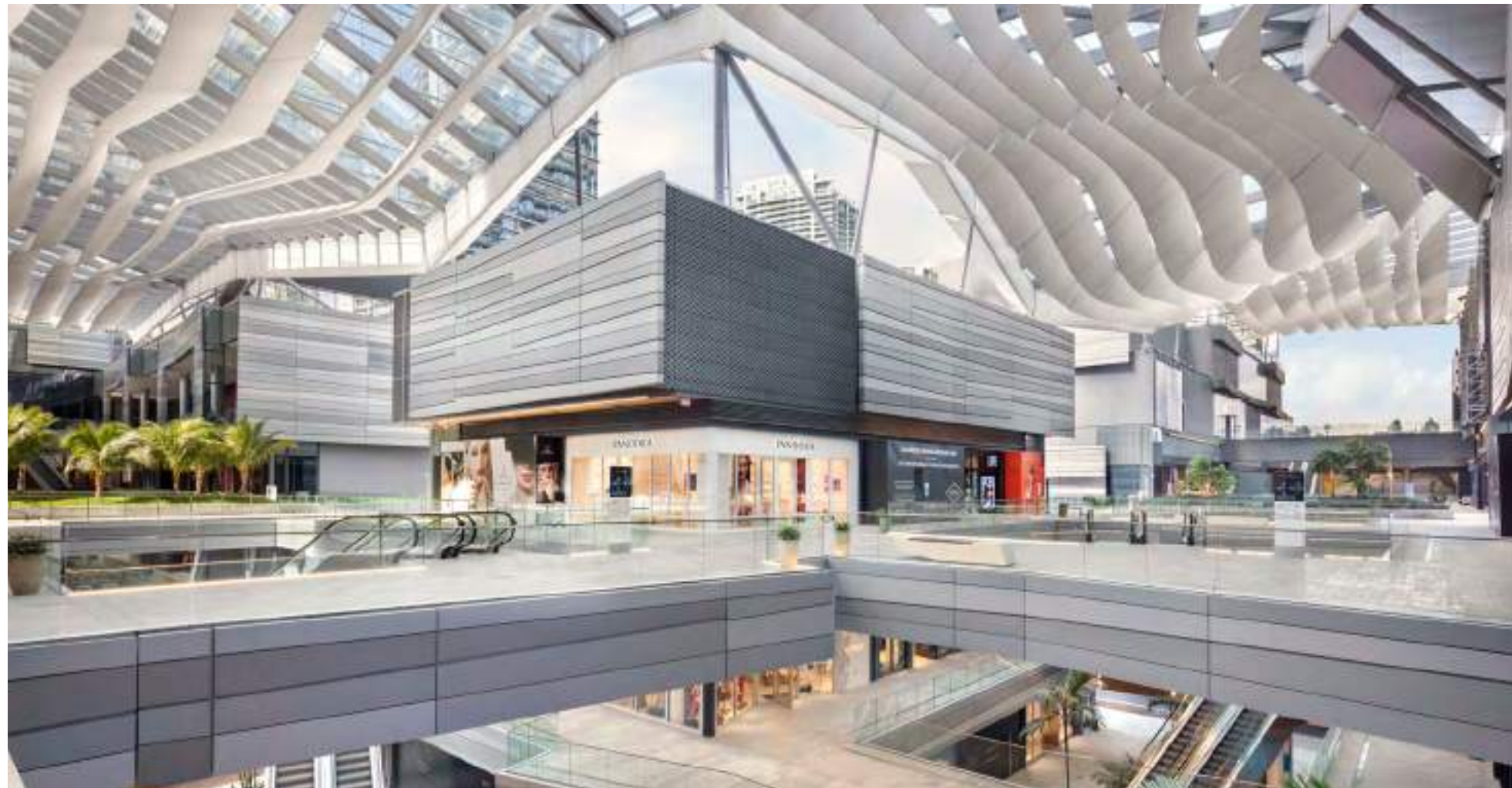
Brickell City Centre, Miami, Florida
